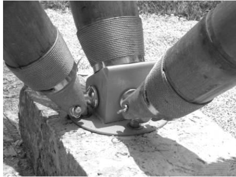
Image 28: Fixing the canes to the foundation with a metallic profile
