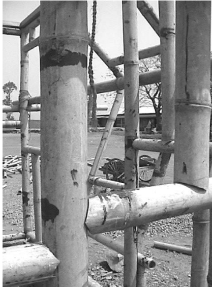
Image 23: Connections in "fish mouth"
