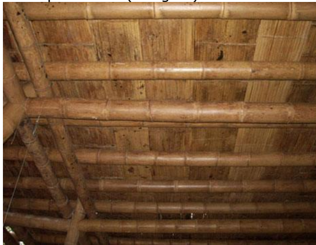
Image 5: „Esterilla” mats, placed above the secondary bamboo beams
