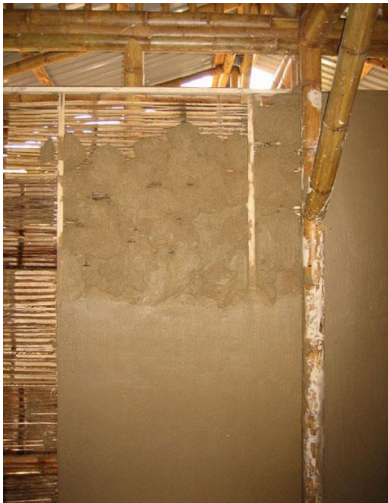
Image 2: Wall made from plastered „esterilla”
