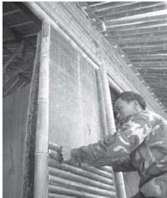
Image 1: Building a wall with horizontal culms
