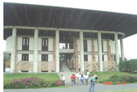
Image 13: Bamboo trusses are used to build a roof structure(Guyaquil, Ecuador, arch J. Morán)
