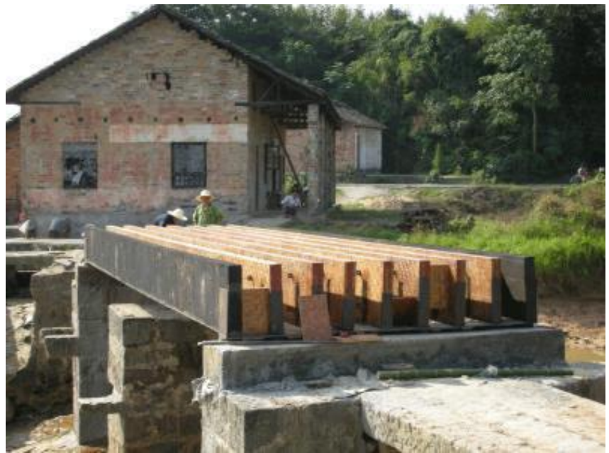
Image 17: Bridge built using GluBam
