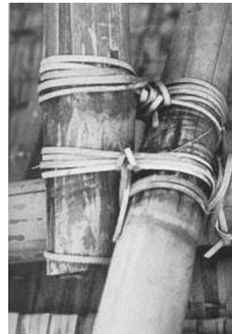
Image 22: Connections using bamboo strips
