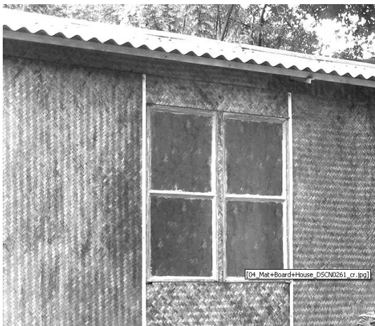
Image 16: The modular bamboo mat board house at IPIRTI
