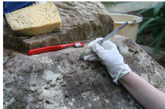
*Image 4: Coats of biocide applied on pedestal and careful cleaning of natural openings of travertine*
