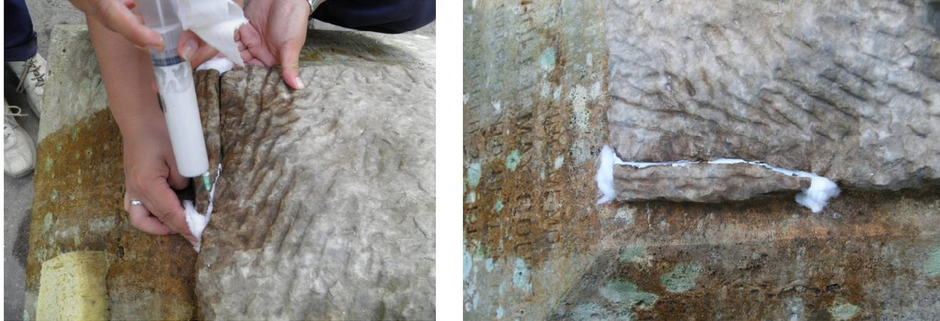
*Image 6: Cracks filling after careful cleaning*
