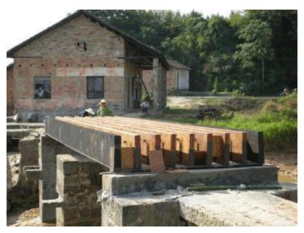
Image 17: Bridge built using GluBam
