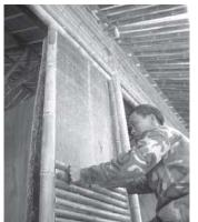
Image 1: Building a wall with horizontal culms
