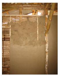
Image 2: Wall made from plastered *"esterilla"*
