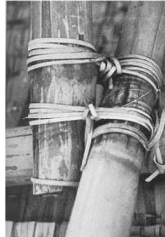
*Image 22: Connections using bamboo strips*
